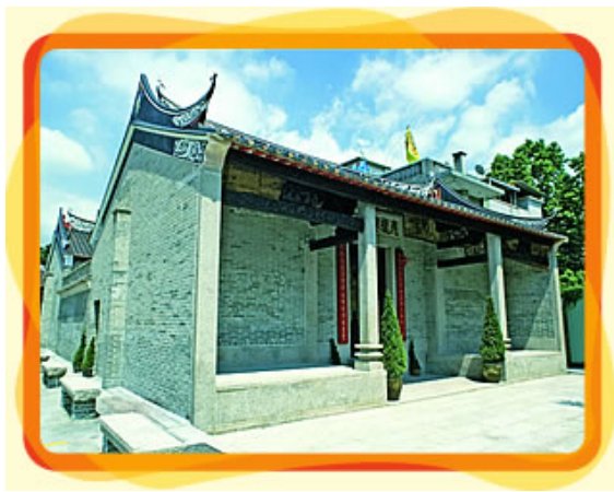
Liu Ying Lung Study Hall after renovation.
