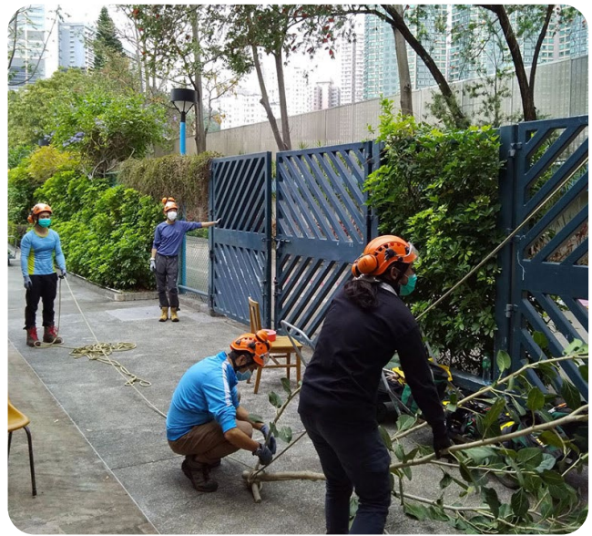
Trainees use a rigging system to carry the pruned branches onto the ground safely during the training course.
