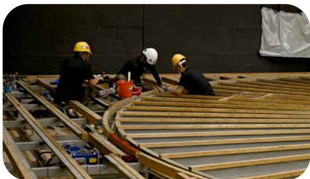
The wheels of the stage wagon and the revolve have been replaced in the Auditorium of the Kwai Tsing Theatre, enhancing the system's stability.
