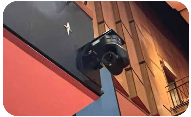
4K remote-controlled cameras and live streaming systems have been installed in the Kwai Tsing Theatre and Tsuen Wan Town Hall, enabling online programmes to be presented in 4K resolution and performing groups to create multi-angle 4K archives.
