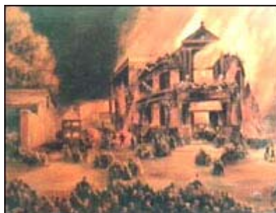
The Theatre Royal in Exeter is destroyed by fire.
